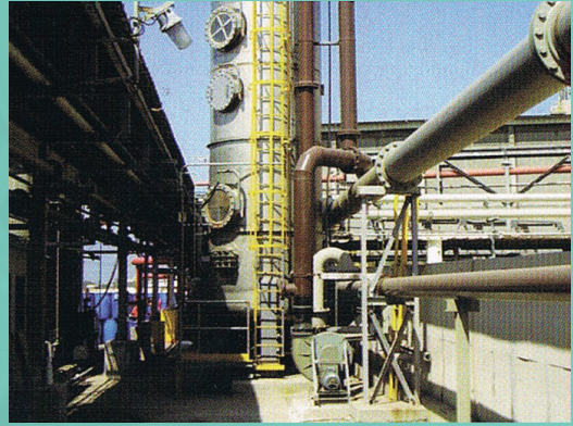
Two-step bio-trickling filter (BTF) purifying polluted air in a sludge treatment plant
