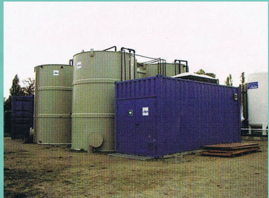
Combined, biological-physico-chem. treatment plant for treatment of complex industrial groundwater
