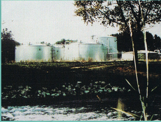
Anaerobic-aerobic Plant for biotreatment of toxic pulp mill effluents
