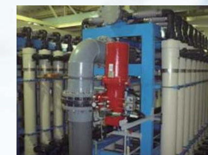
Seawater Desalination (for RO pretreatment) Capacity: 2,700m 3 /d Location: Ehime, Japan Operation start: Sept. 2003
